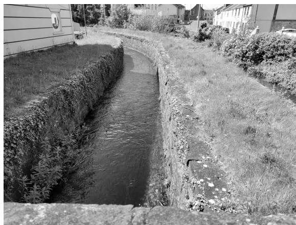
Figure 1: Example of a “mill race” or “mill run” that was used to provide continuous water power to mills (image: author).
